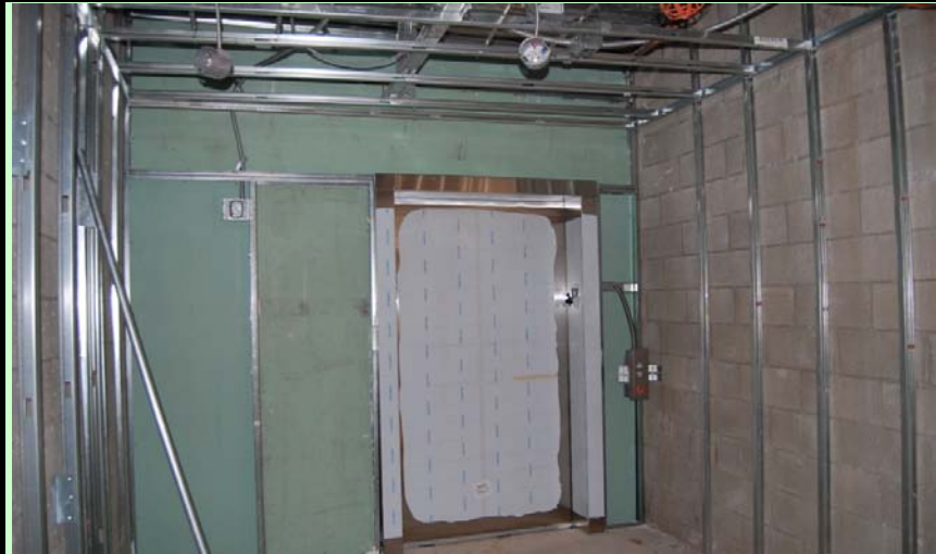
Interior: Ongoing progress with the elevator
