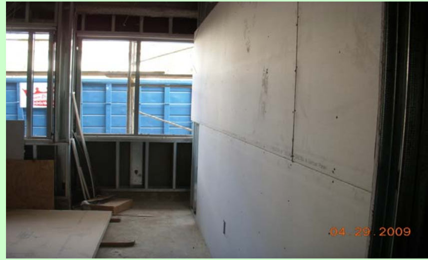
Interior: Drywall underway
