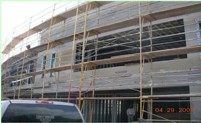
Exterior: Densglass exterior skin underway. Followed by waterproofing and Jerusalem stone
