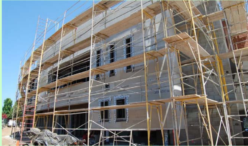
Exterior: Densglass exterior skin underway. Followed by waterproofing and Jerusalem stone
