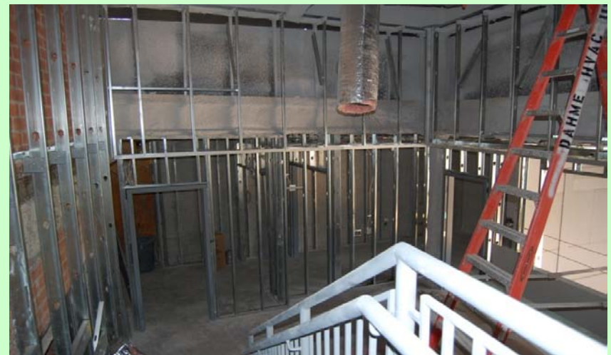
Interior: Upper library mezzanine underway
