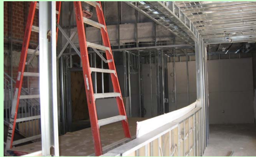
Interior: Library @ 3rd floor
