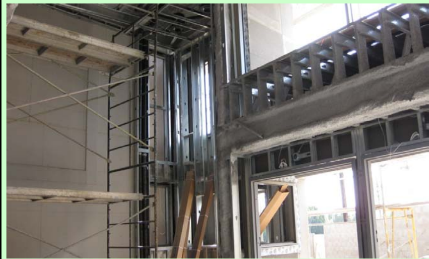
Interior: General progress
