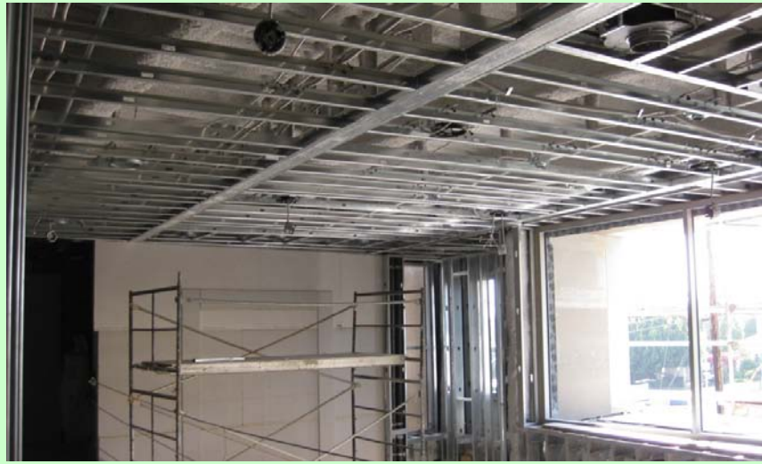
Interior: Waiting to install 2nd layer of drywall
