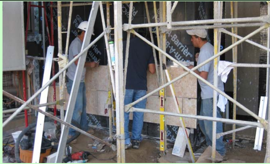
Exterior: Jerusalem stone install underway at tower!
