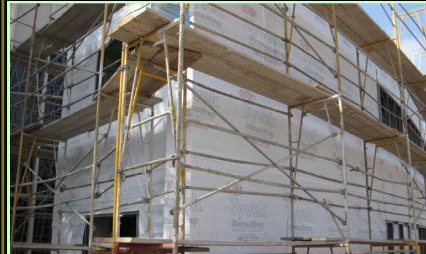
Exterior: General progress with Tyvek wrap
