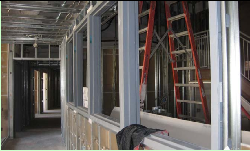
Interior: Library @ 3rd floor - window frame installed
