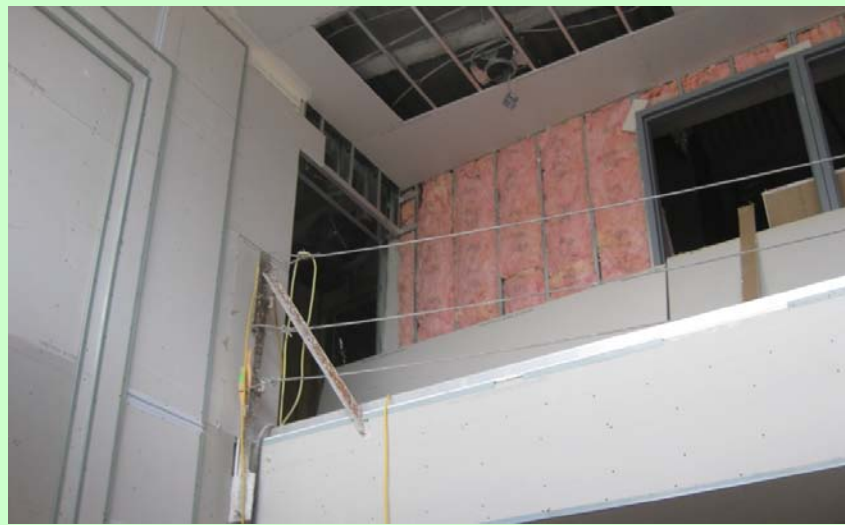
Interior: Library @ 3rd floor - Insulation in walls
