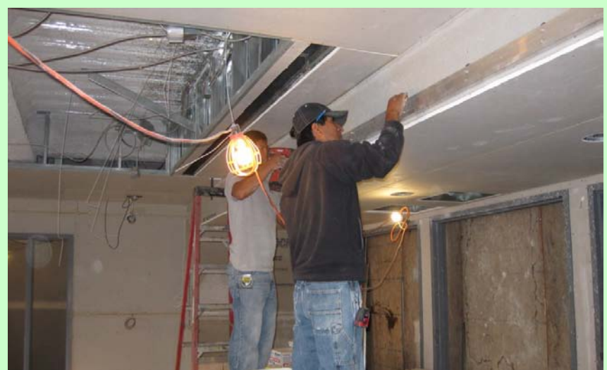
Interior: General progress @ lobby
