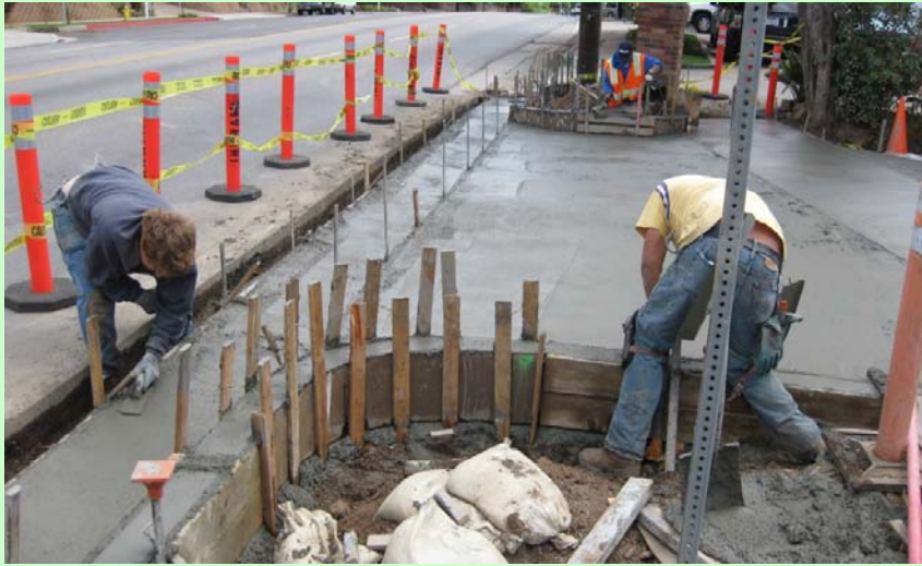
Exterior: Driveway / Street / Sidewalk work @ Sunset Blvd
