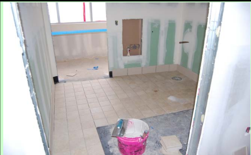
Interior: 2nd floor restroom tile underway
