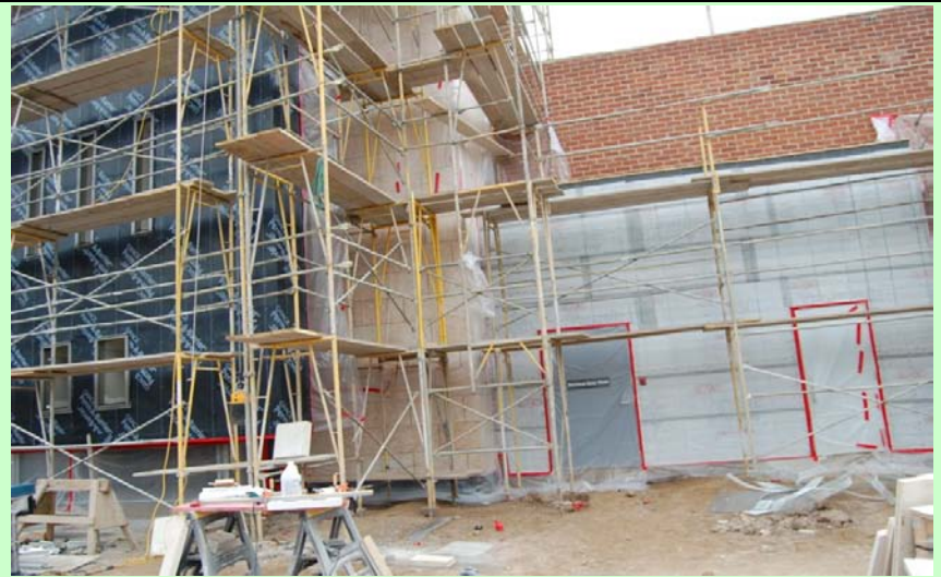
Exterior: J-Stone installation almost complete at tower
