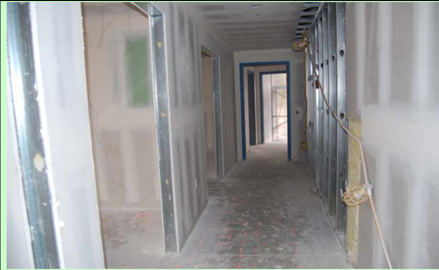
Interior: 2nd floor corridor
