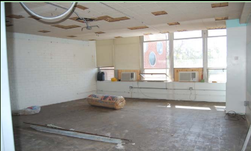
Interior: 2nd floor student lounge has started!
