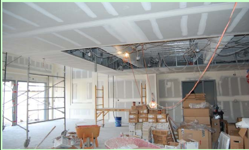
Interior: Lobby taped - ready to prime
