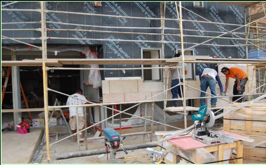
Exterior: Jerusalem stone continues on the main portion of the building now that it has finally arrived! Mazeltov!
