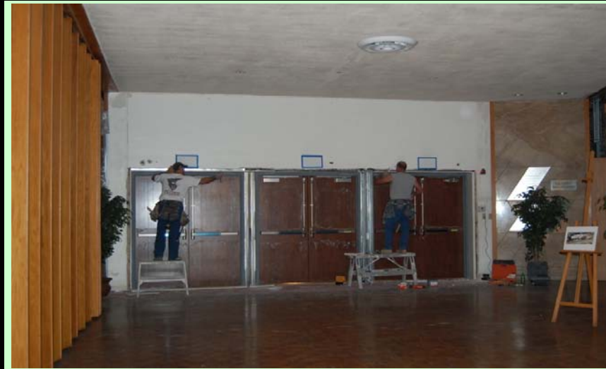
General Progress: Doors into the new wing now visible!
