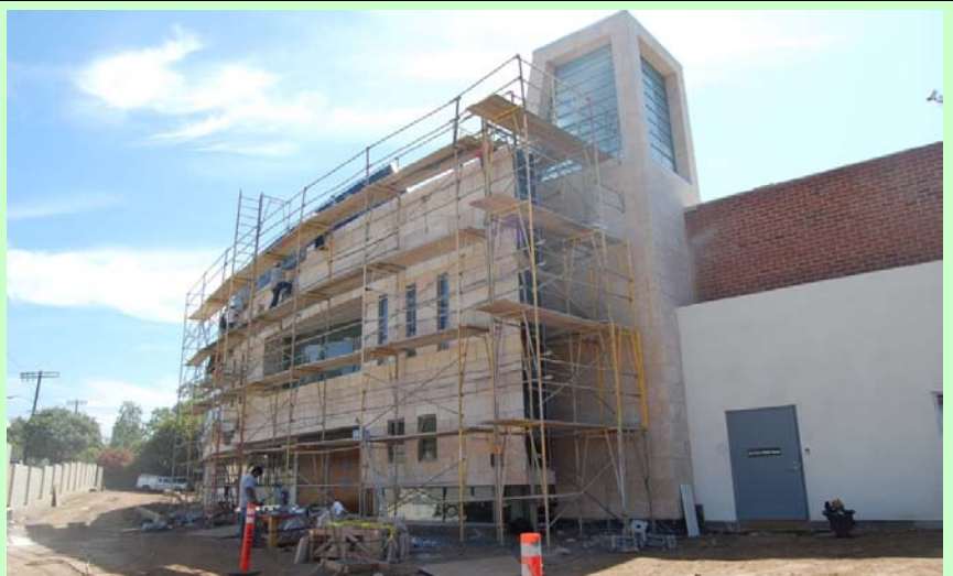
General Progress: J-stone progress
