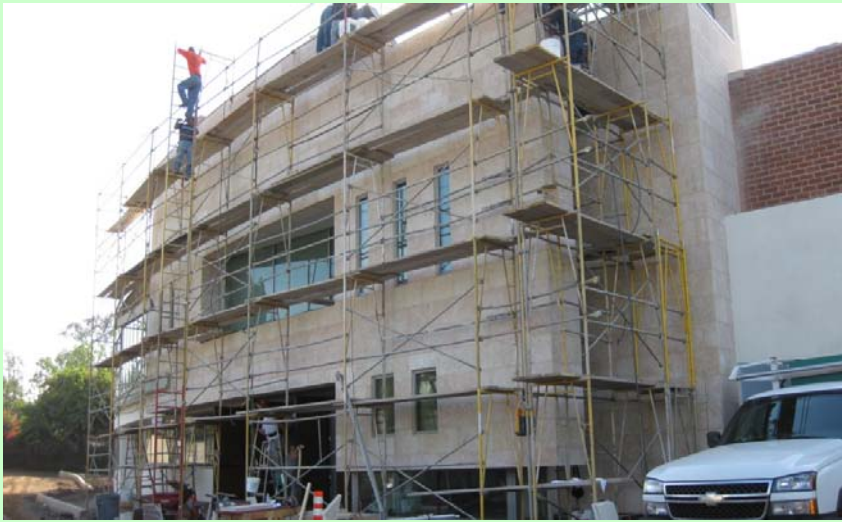
General Progress: Grouting the stone
