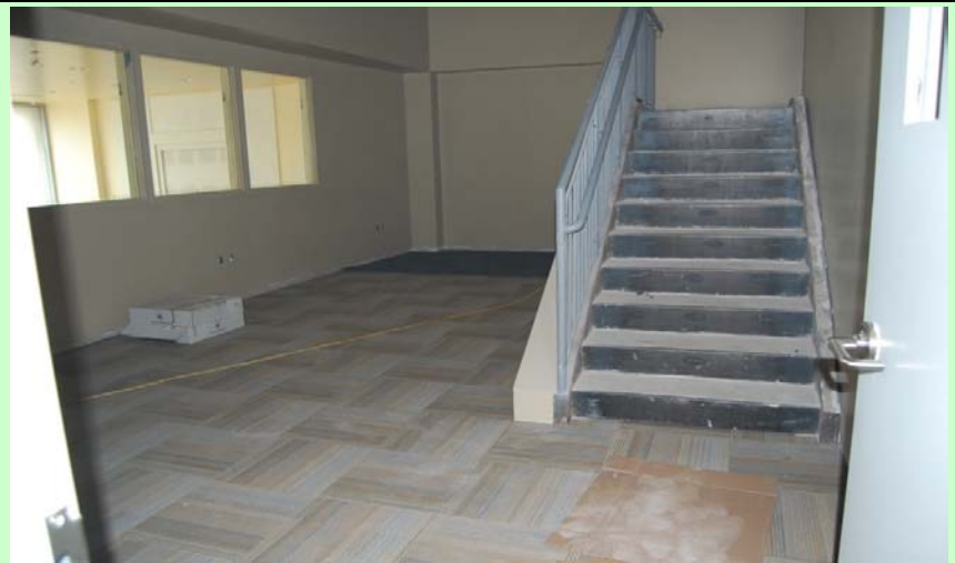
General Progress: library carpeted
