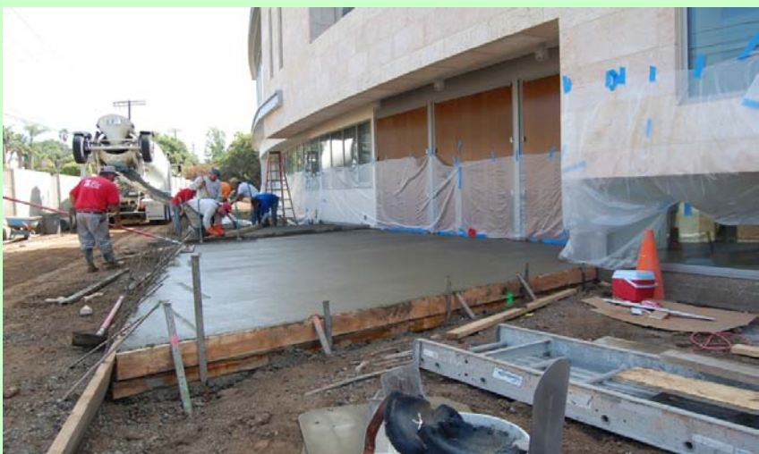
General Progress: entry concrete poured
