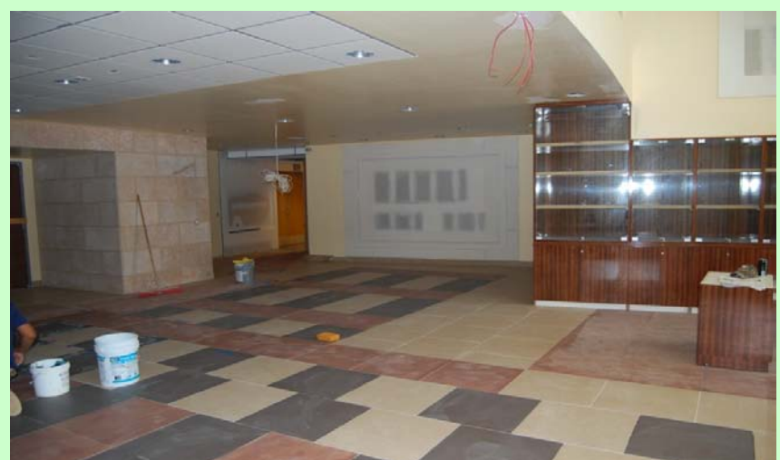
General Progress: interior lobby tile almost complete and grouted
