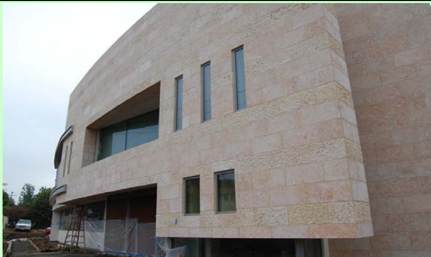
General Progress: stone complete, scaffold removed
