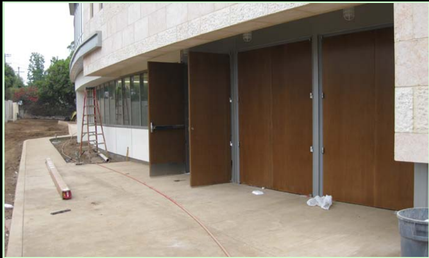
General Progress: Concrete pathways and at entry complete
