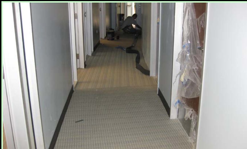
General Progress: Carpet in offices and corridors substantially complete
