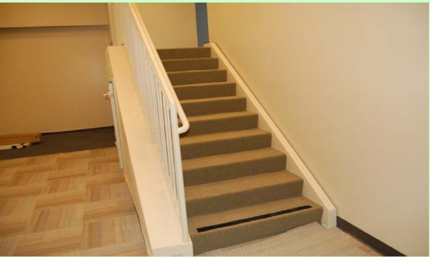
General Progress: Library mezzanine carpet @ stairs
