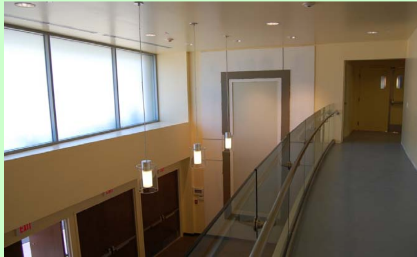
General Progress: Interior. Flooring down (seam welding and base pending). Clean up by JPI underway
