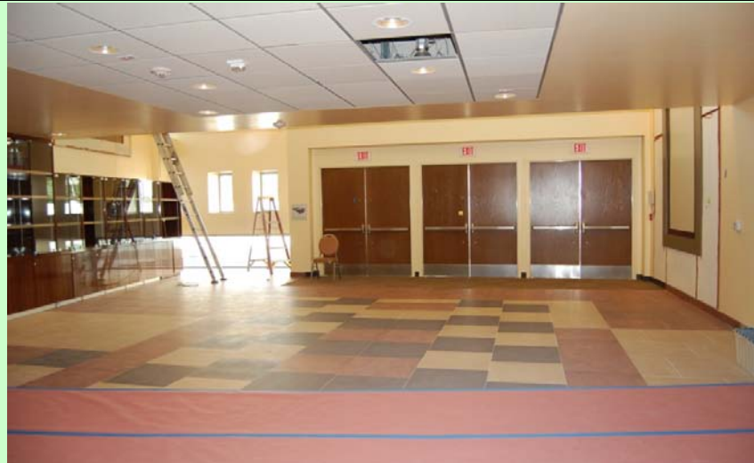
General Progress: Lobby "punch" underway
