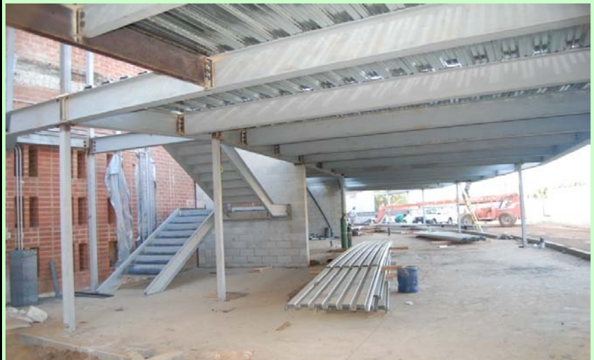
Exterior: Structural framing and metal decking underway
