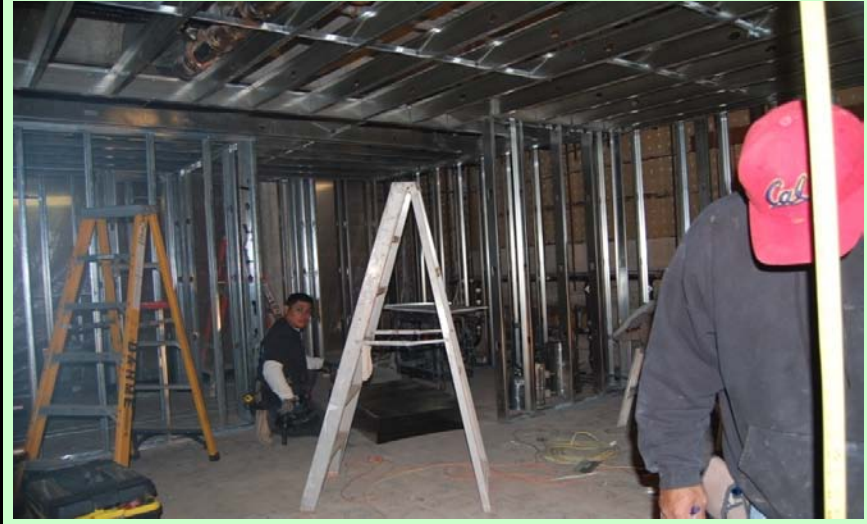
Interior: Woman's bathroom work underway
