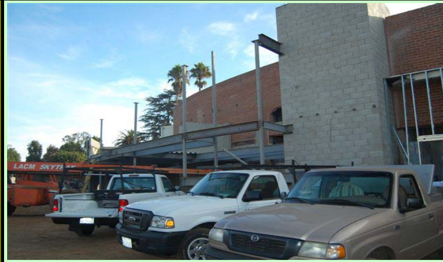
Exterior: Structural framing and metal decking underway
