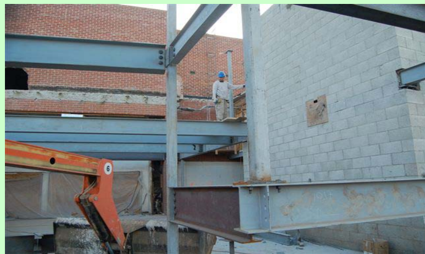
Exterior: Structural framing and metal decking underway
