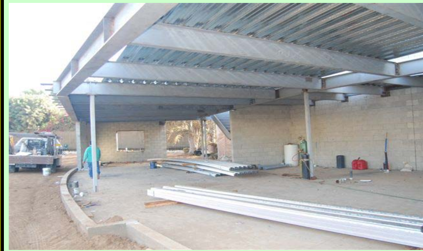
Exterior: Structural framing and metal decking underway
