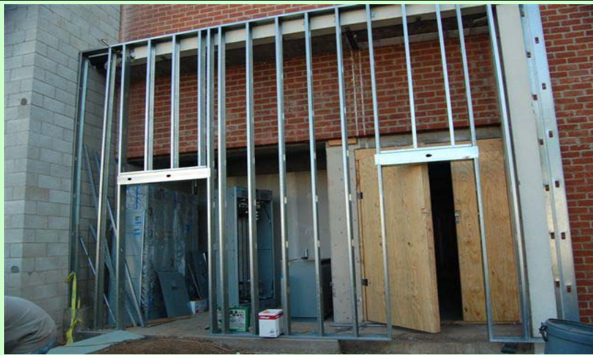
Exterior: Framing @ new entry
