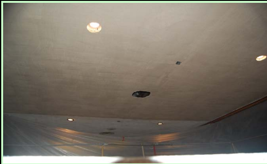
Interior: Klein hall ceiling finished now structural is complete. Finished "rough" to match existing abated finish
