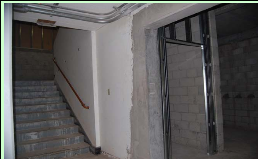
Interior: 1st floor tie in old / new structure
