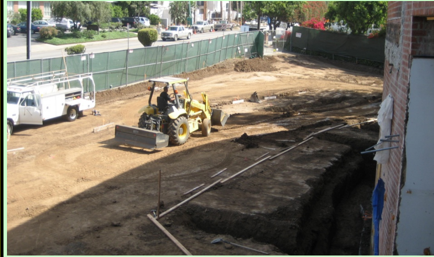
Exterior: Ongoing excavation for footings (part of foundation system)
