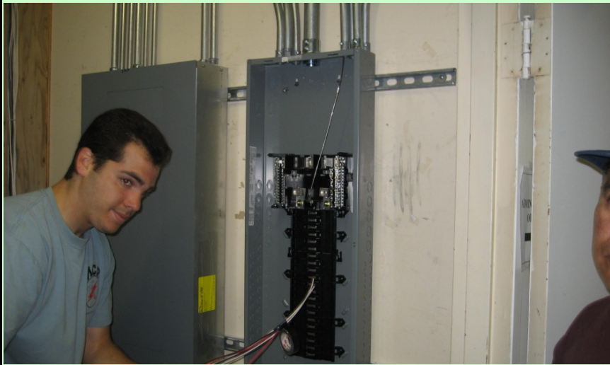
Interior: New electrical panel and wiring for interior tenant improvement area
