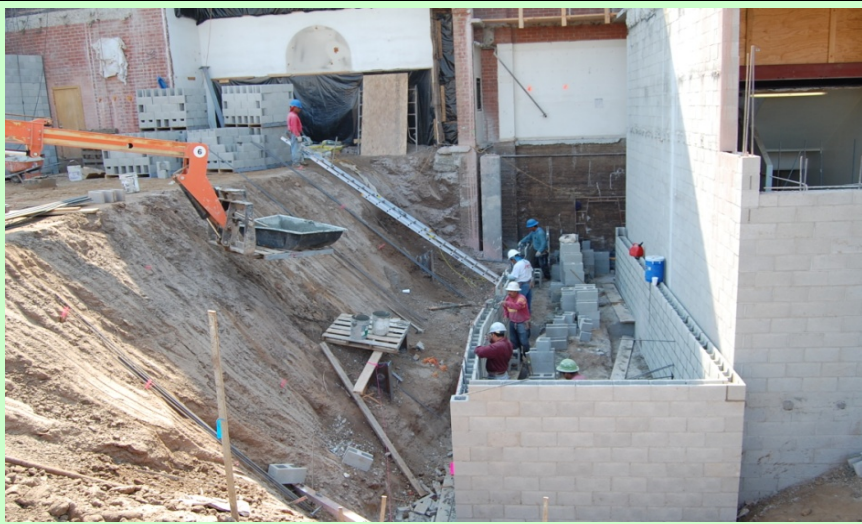
Exterior: Basement CMU walls for elevator shaft underway
