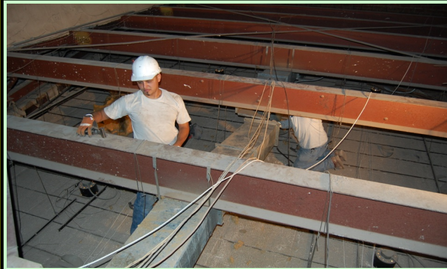
Interior: Ductwork installation underway above sanctuary ceiling
