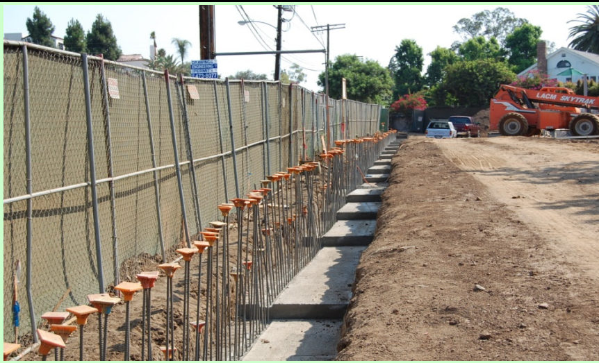
Exterior: Footings poured for Sunset wall.
