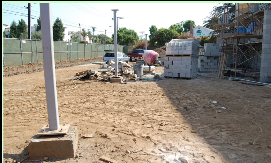
Exterior: Tubular steel columns set in place (but not finished)
