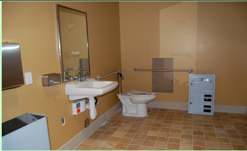
Interior: Bathroom fixtures continue...almost there.
