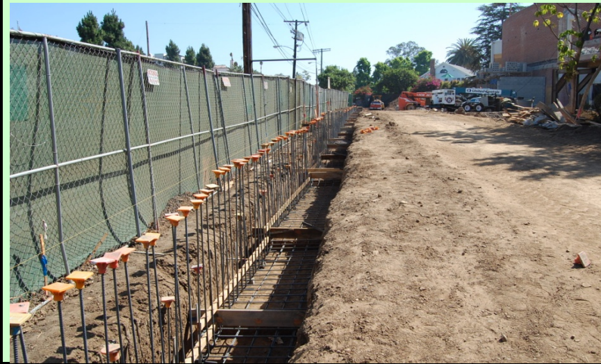
Exterior: Rebar installed for footings for new wall along Sunset .
