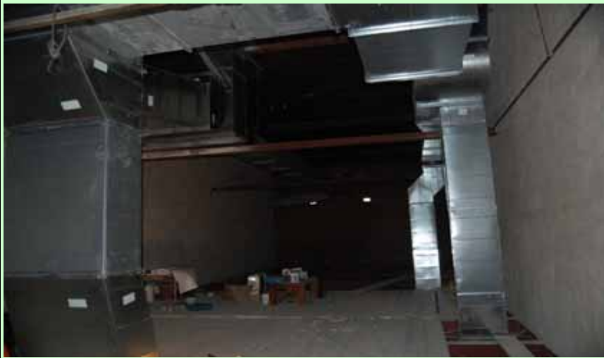
Interior: General progress photo - library / ductwork
