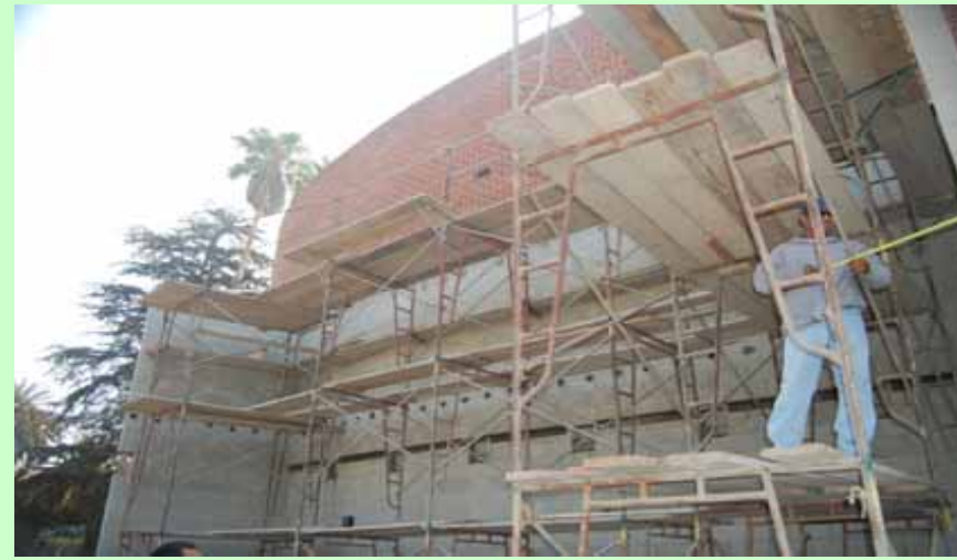
Exterior: Scaffold erection
