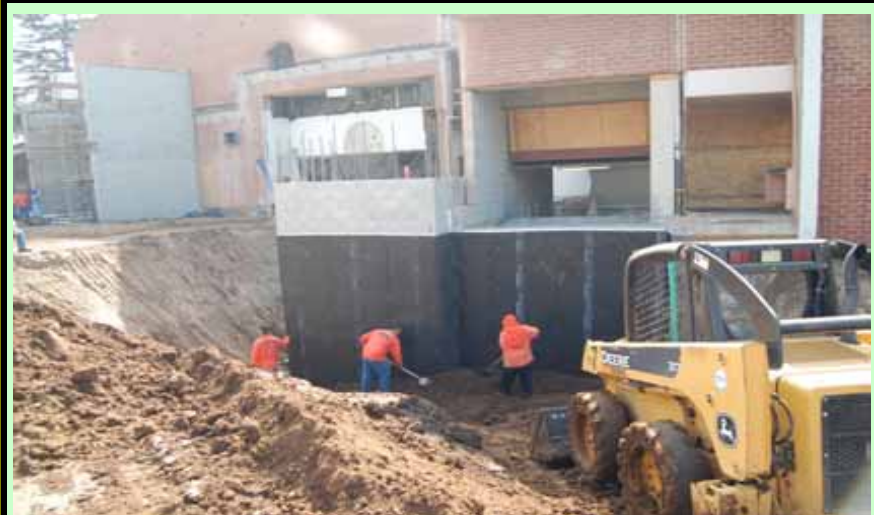
Exterior: Below grade waterproofing complete, back-fill of dirt underway
