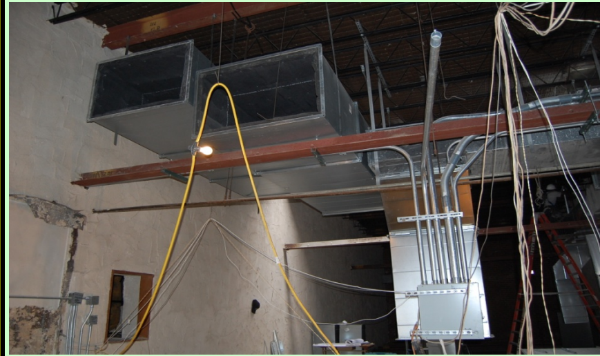
Interior: Ductwork installation underway
