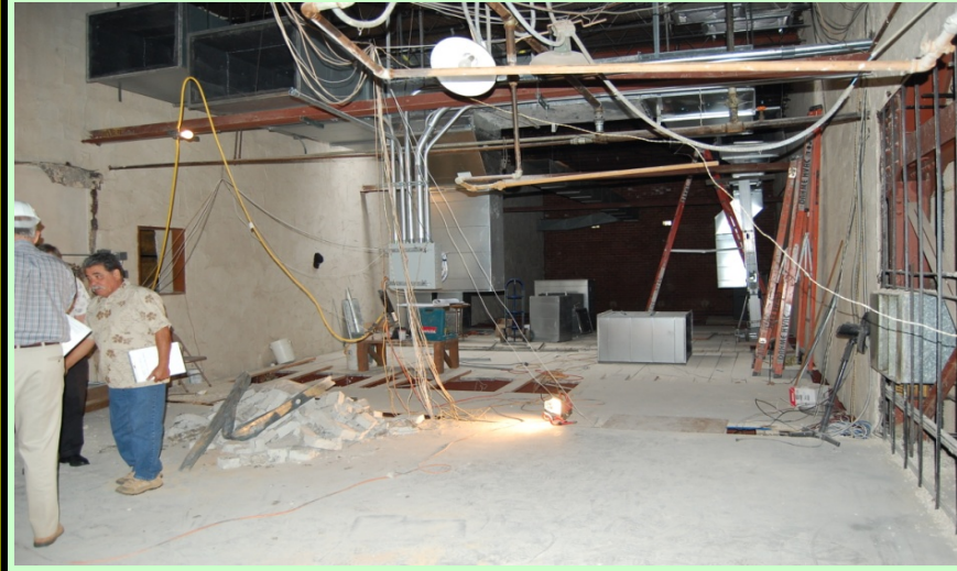
Interior: Inside new library area in foreground.
