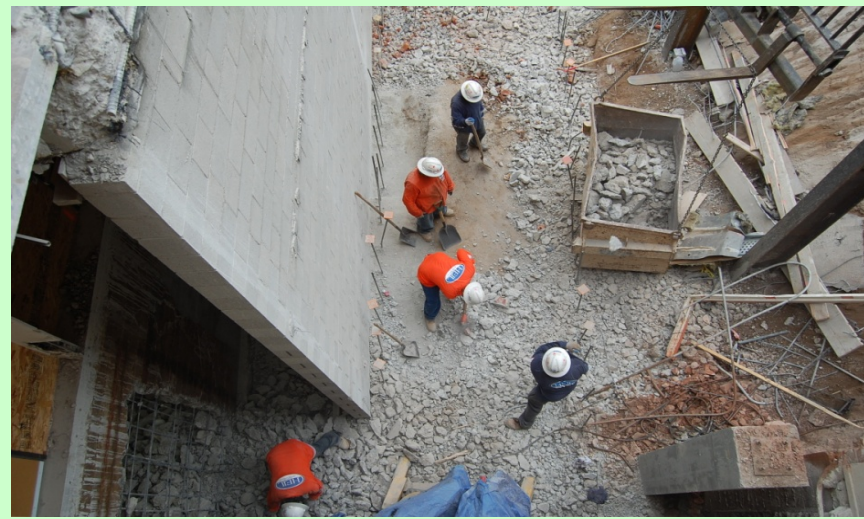
Exterior: Demo and clean up continues
