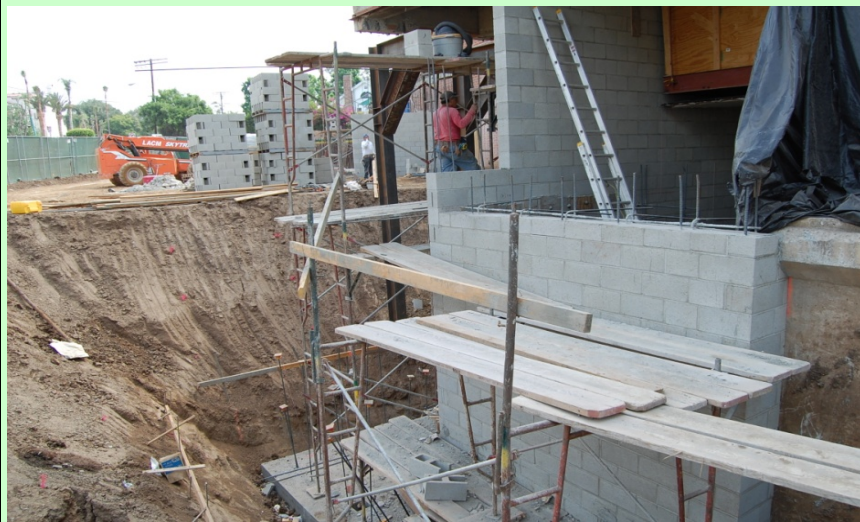
Exterior: Ongoing CMU work
