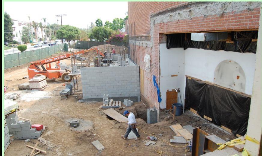
Exterior: Note CMU walls underway.
