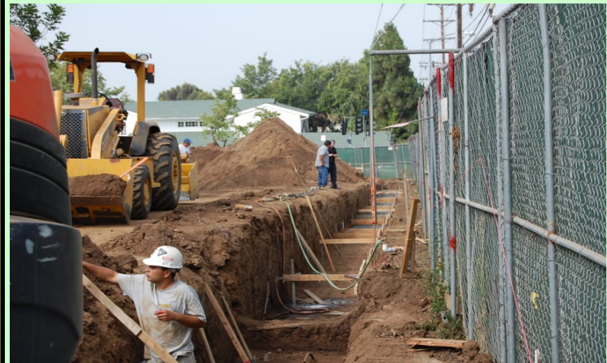
Exterior: Trench for footings for new wall along Sunset has been excavated and forming has started to enable concrete pours.
