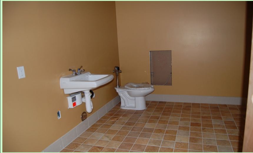
Interior: Bathroom fixtures installed! Almost done!
